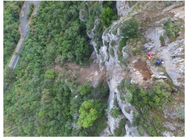
Figure 4. Inspection and scaling works
