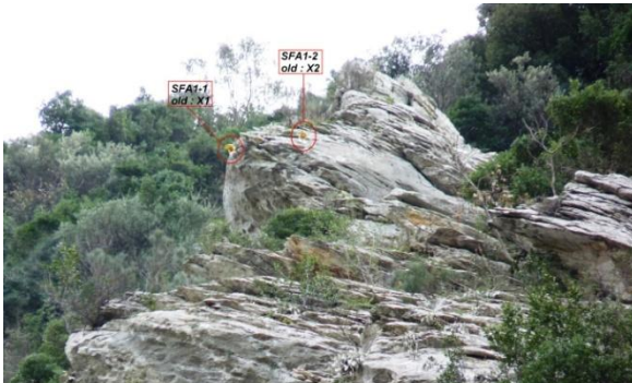
Figure 6. Prisms installed in special focused area SFA1.
